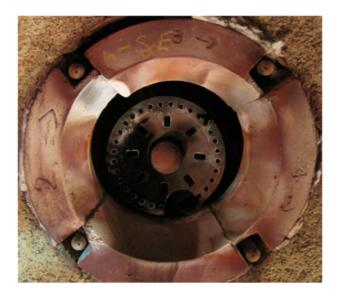
Figure 15 Burner tile segments improperly aligned.
