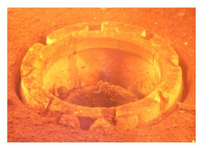
Figure 16 Burner tile installed upside down.
